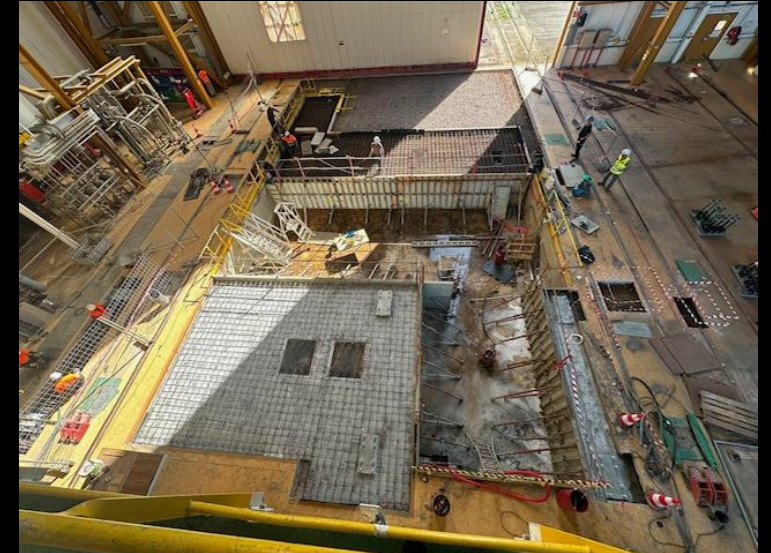
Vega Assembly Building
