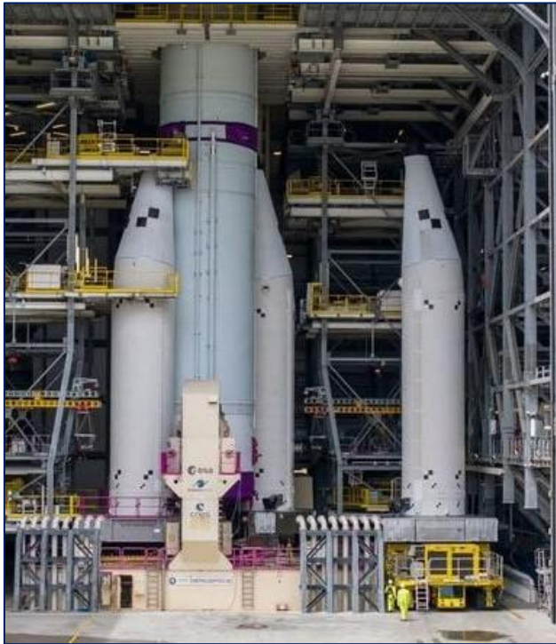
Installation of 4 boosters on central core
