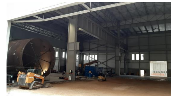
New 4562 Building under construction
