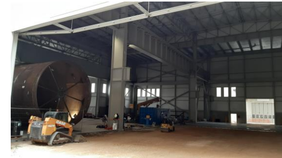
New 4562 Building under construction
