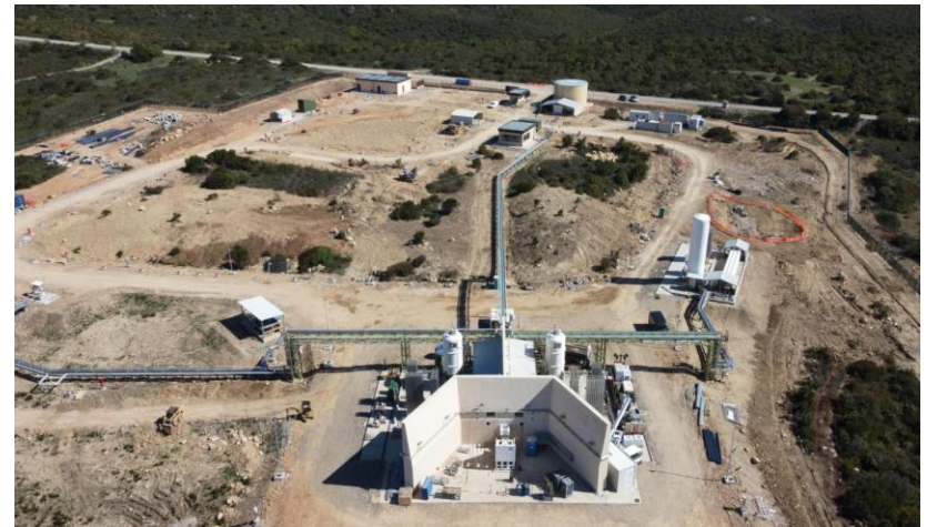
SPTF facility under construction in Sardinia
