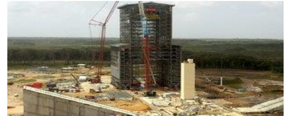
Ariane 6 mobile gantry in construction
